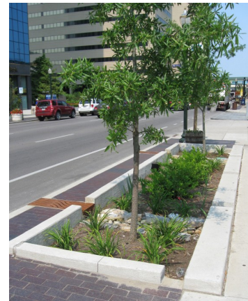
Pictured above are examples of naturalized stormwater planter systems that collect stormwater runoff.
