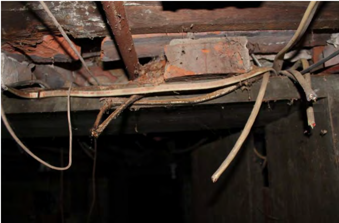
Photo 7 – View of assumed asbestos-containing braided wire insulation in the basement.
