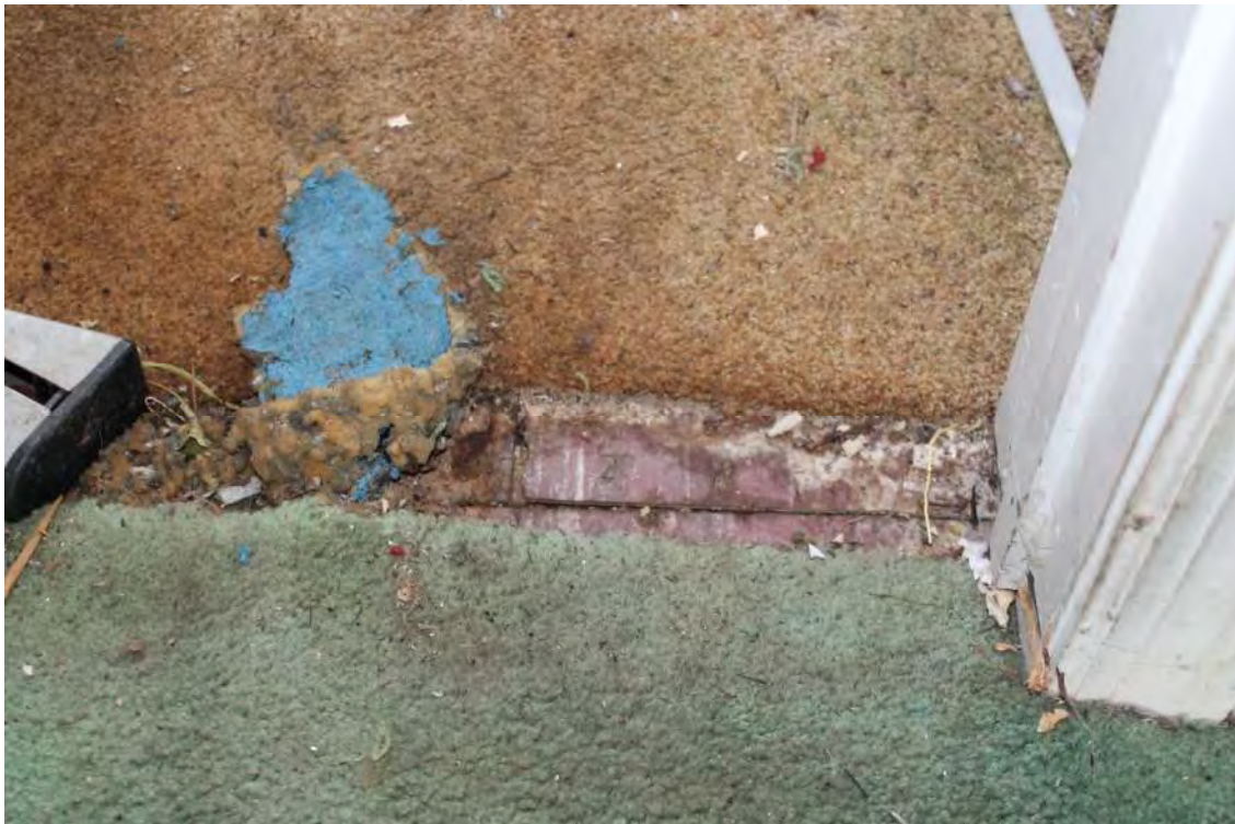
Photo 10 – View of asbestos containing 9 x 9 maroon floor tile and associated black floor tile mastic under carpet in the second-floor apartment.
