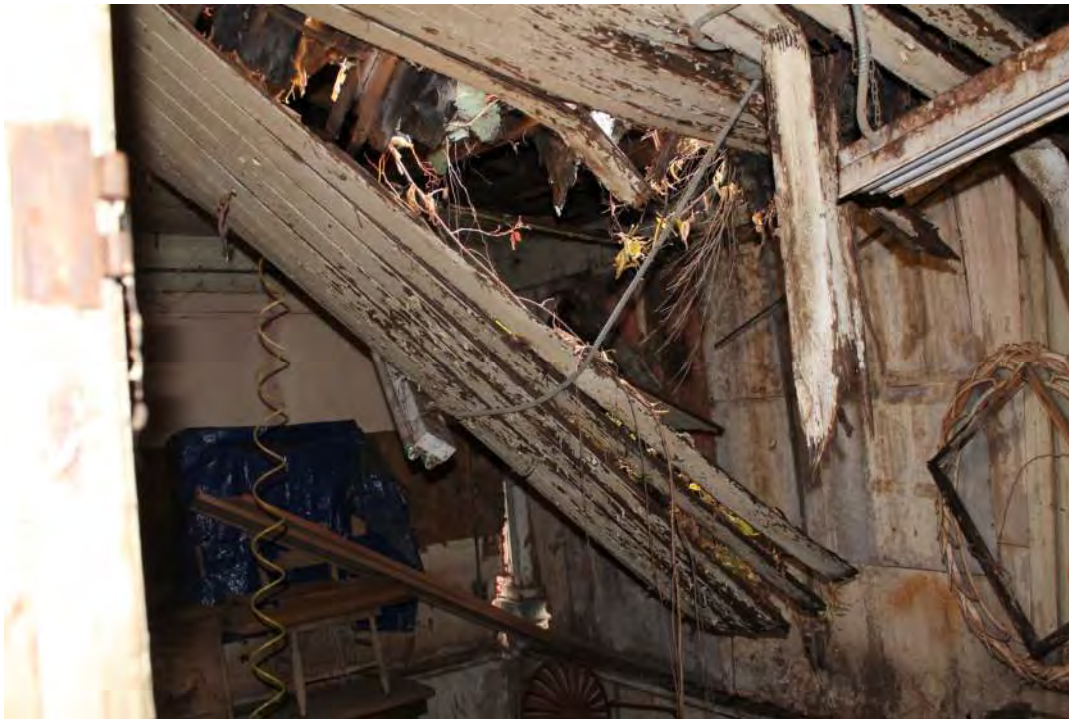
Photo 2 – First floor ceiling collapse in the back of the first floor.
