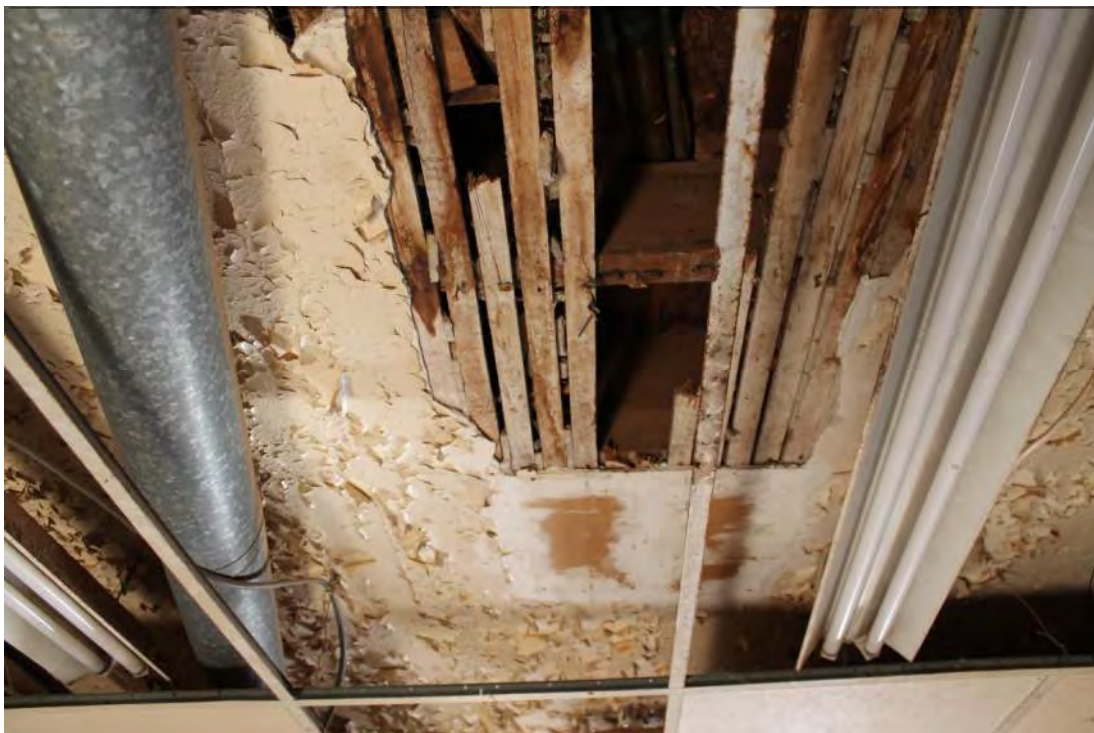
Photo 5 – View of asbestos-containing ceiling plaster skim coat on the first floor workshop area.
