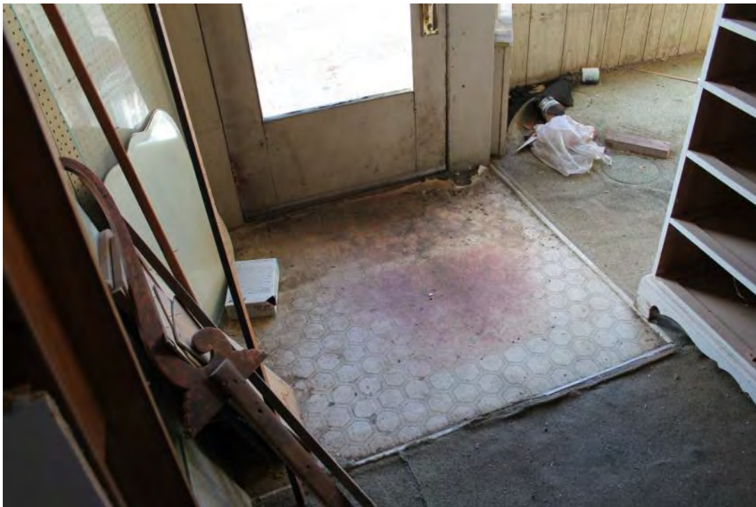
Photo 3 – View of asbestos-containing sheet vinyl floor at entry. 9 x 9 floor tile located below sheet vinyl.
