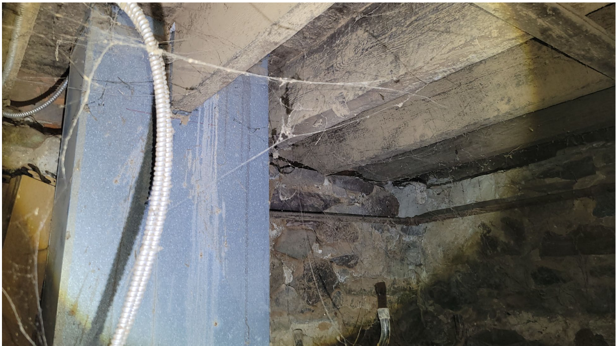
Photo 12: Reroute ductwork around joists, or install a header to support the joist. Remove joist hangers from duct work. Do not bear joists on ductwork.
