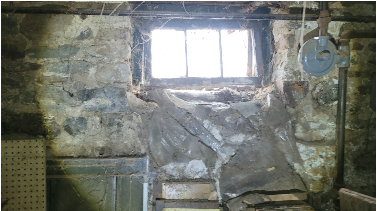
Photo 14: Seal all cracks and voids in foundation wall with non-shrink grout, epoxy sealant, or parging.
