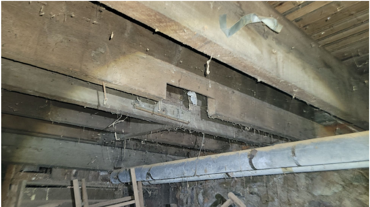
Photo 48: Sister 2x10 joist at all cut floor joists. Extend past 24" with #8 screws @ 12" o.c.
