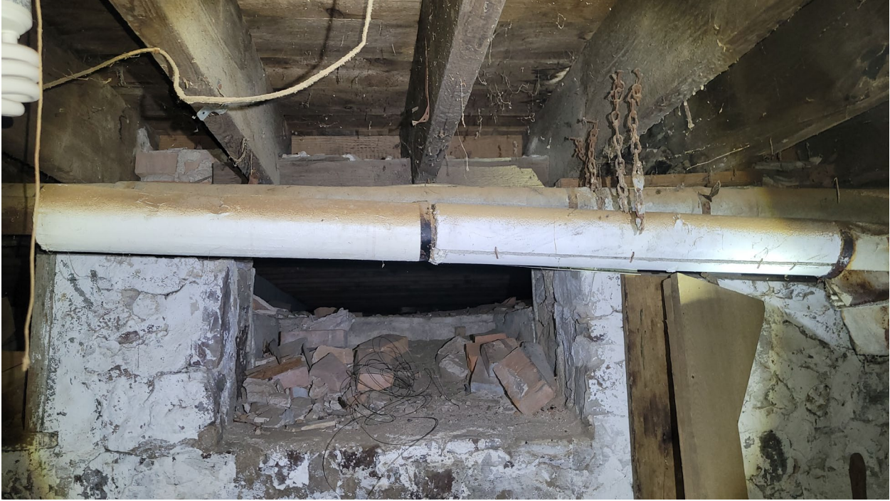
Photo 31: Pipe coverings could have asbestos in them. It is recommended to either test the insulation for asbestos, or have removed by an asbestos remediation professional.
