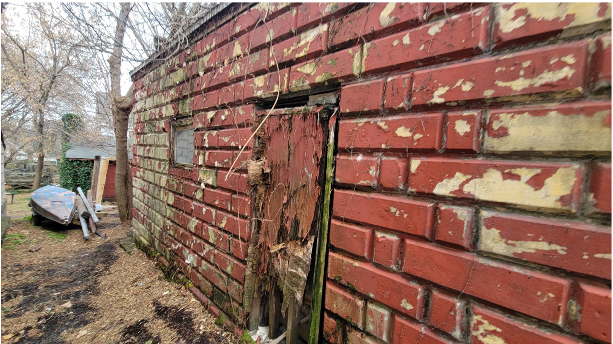
Photo 152: Remove all rotted wood from exterior and infill opening to be watertight.
