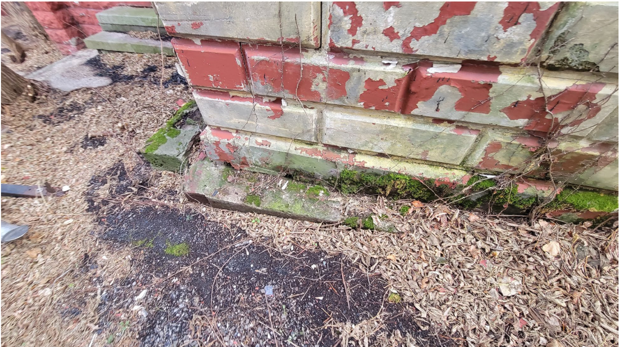
Photo 158: Clean all moss off of foundation blocks and repoint cracks or fill with an epoxy sealant.
