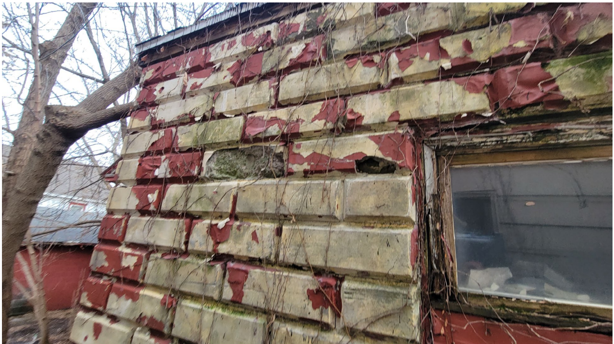
Photo 156: Repoint face of exterior block to prevent moisture degradation.
