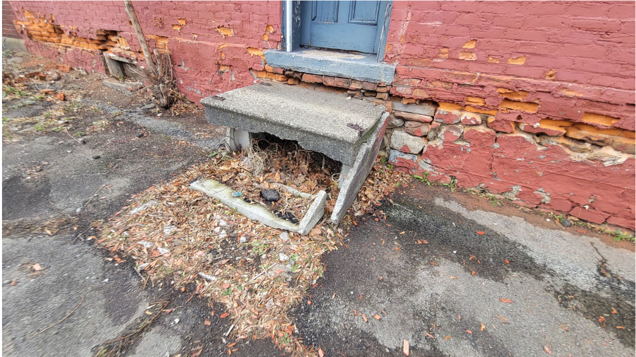
Photo 173: Remove and replace steps.
