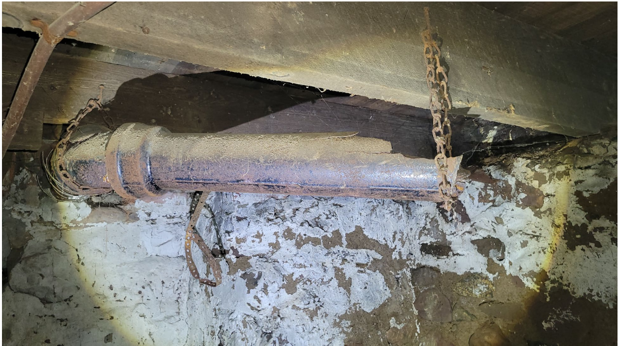
Photo 8: Remove and dispose of all abandoned pipes.
