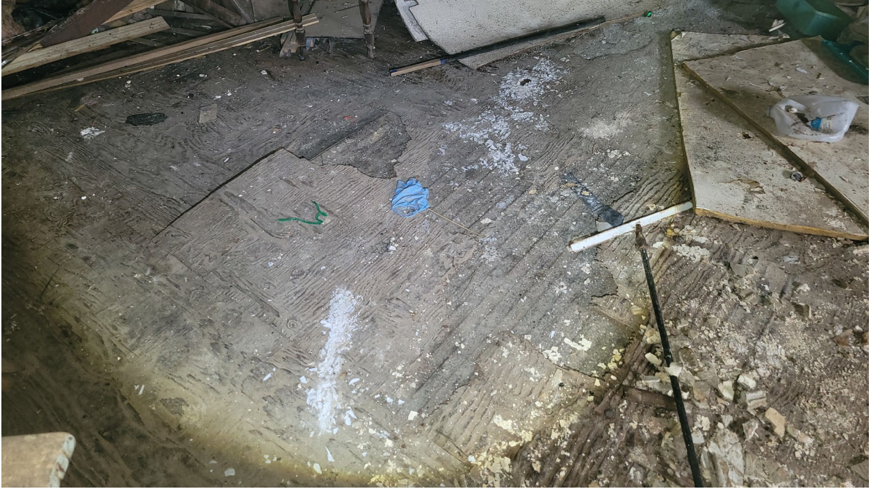
Photo 89: Remove and replace in kind existing subfloor,
