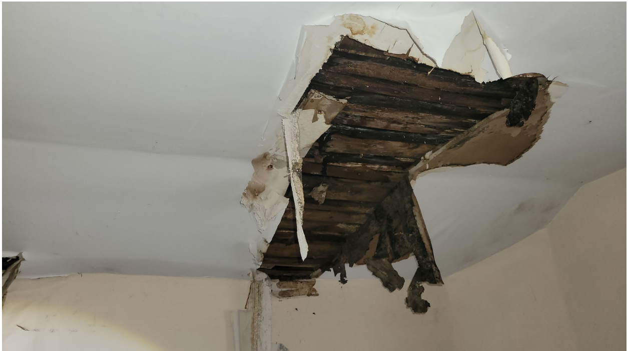
Photo 116: Remove and replace all existing ceiling lathe that is water damaged.
