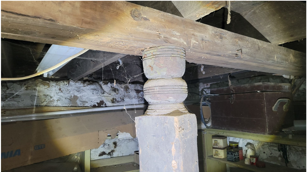
Photo 6: This post needs to be replaced with a steel jack stud.
