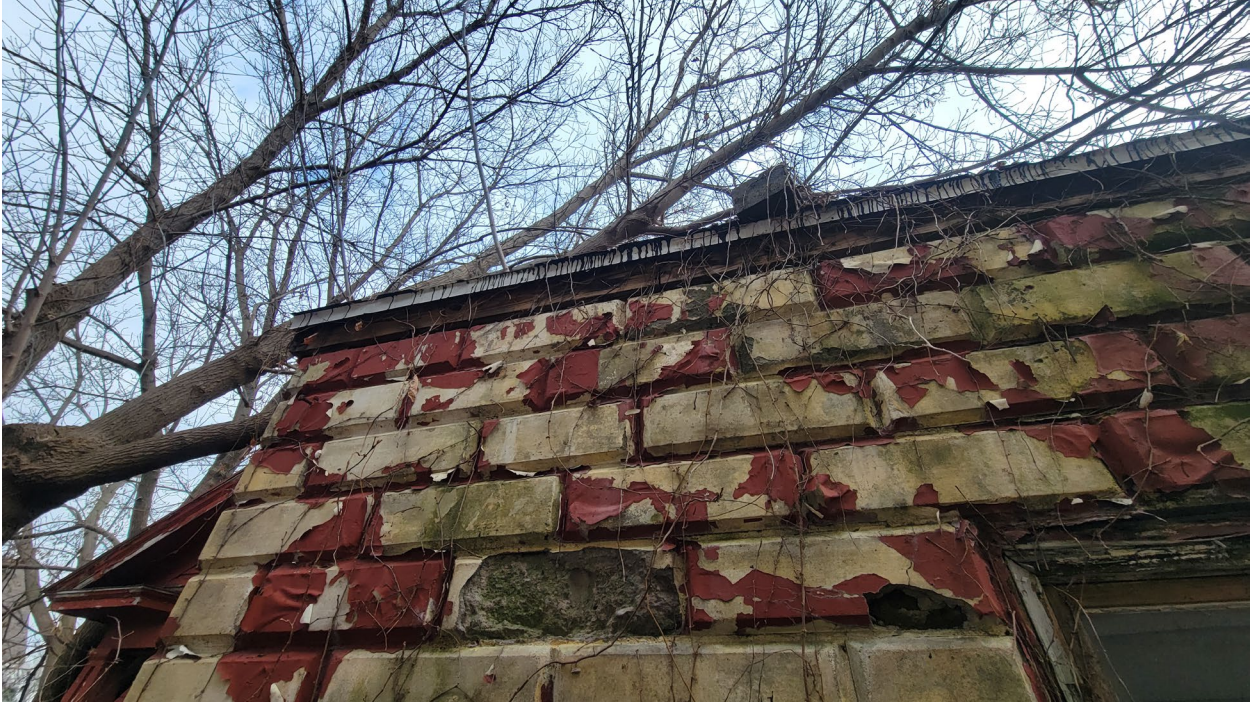
Photo 157: It is recommended to install gutters and replace the rotted eave plate with new pressure treated lumber in kind.
