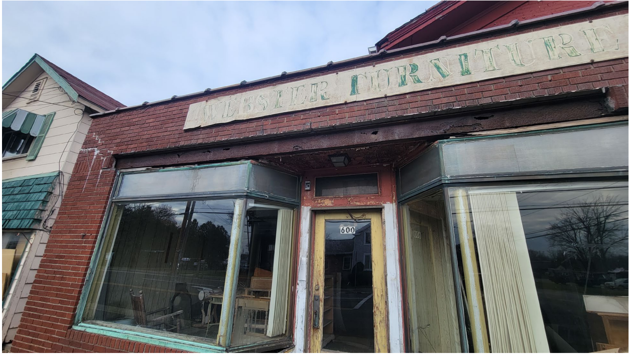
Photo 145: Steel lintel needs to be replaced, see note 8.
