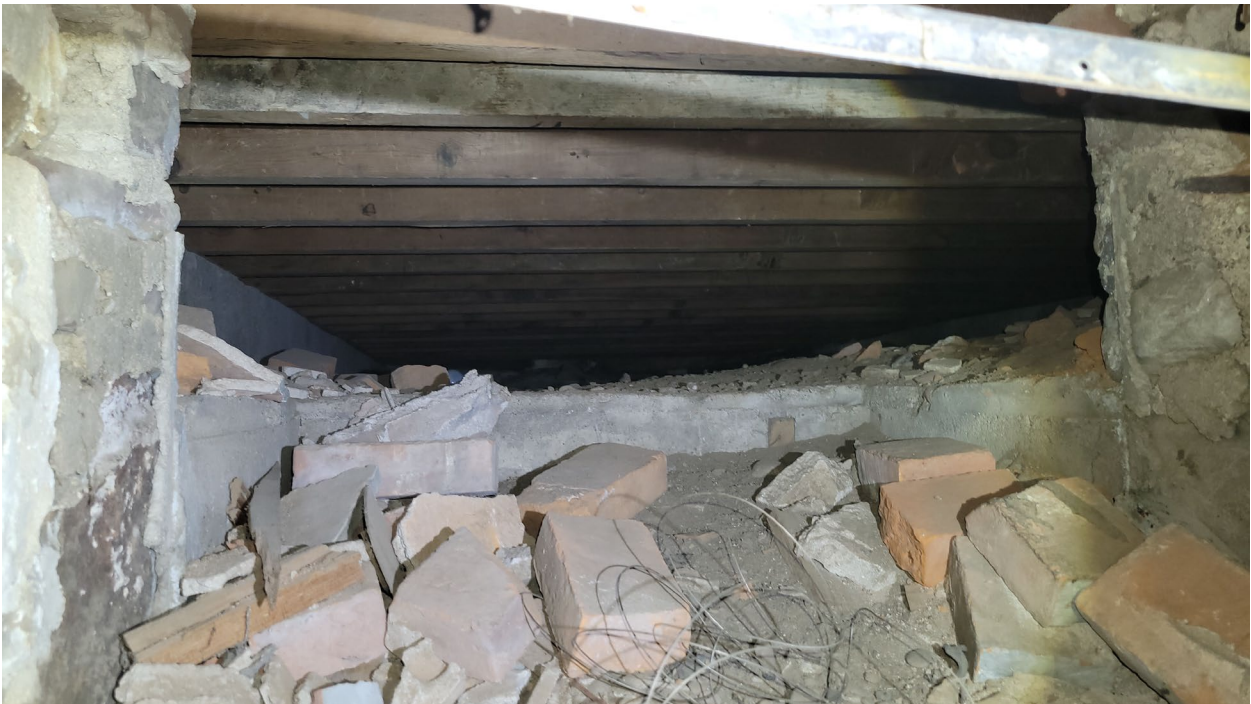
Photo 32: It is recommended to run a dehumidifier in the crawl space to prevent any moisture or mold build up in this area.
