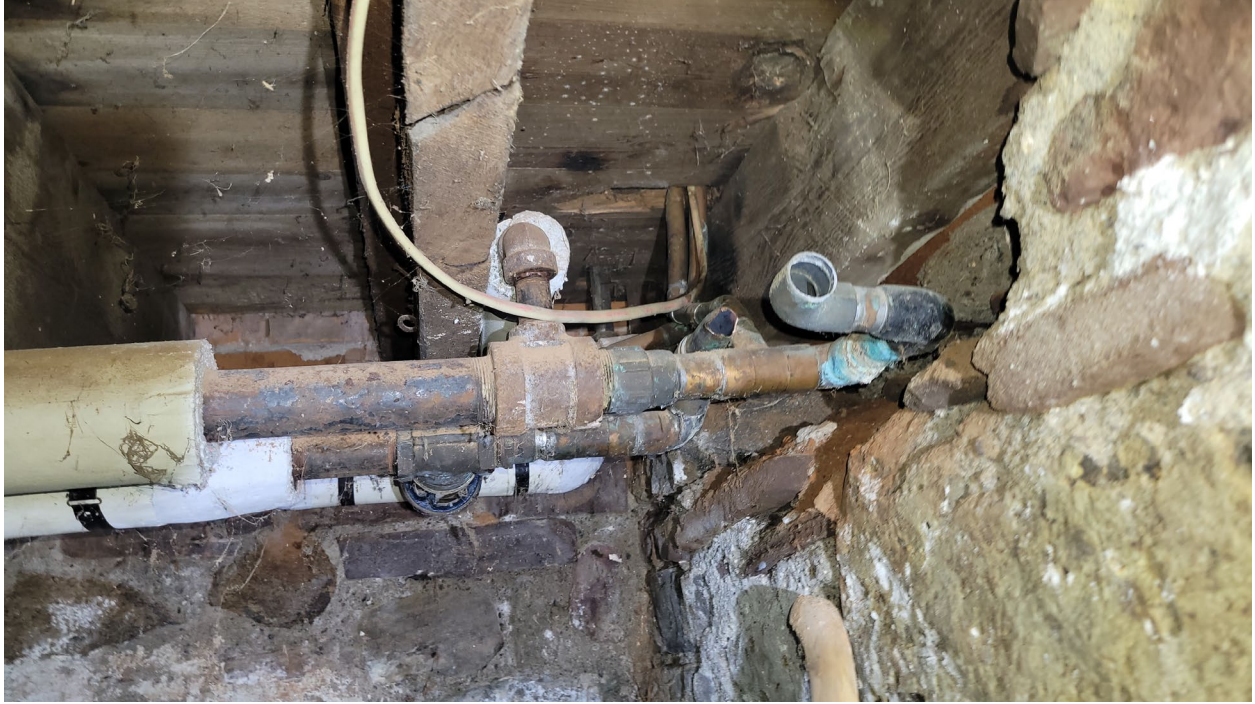
Photo 55: Cap or remove all abandoned piping.
