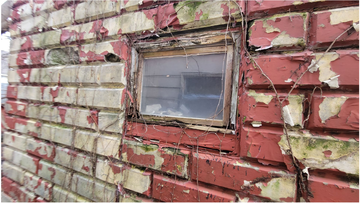
Photo 155: Recommended to replace window with glass block.
