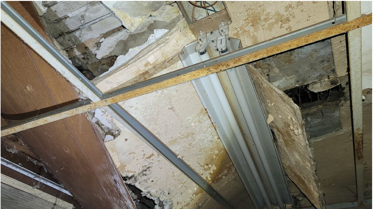
Photo 72: Remove all fallen or delaminated ceiling panels.
