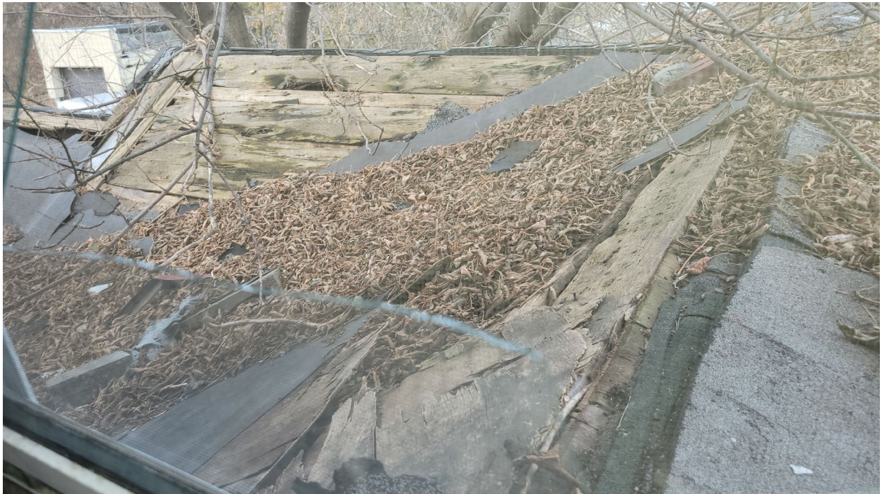
Photo 120: Roof needs a full tear off and replacement. Existing rafters that are not rotted can be salvaged.
