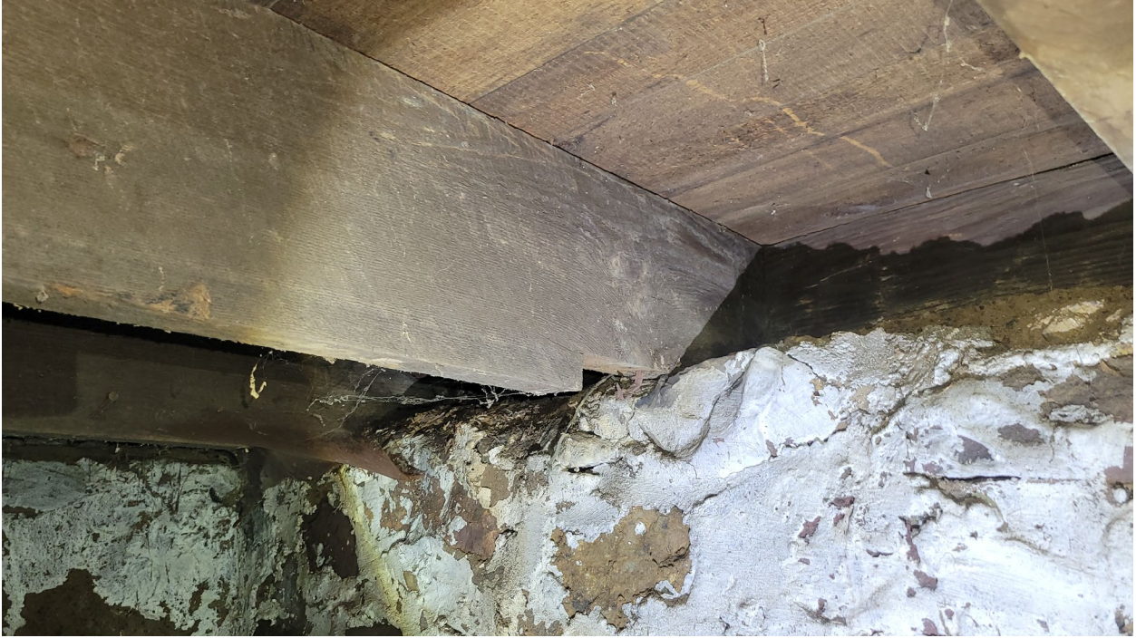
Photo 9: Sister new 2x10 joists to existing framing to properly bear on existing foundation wall.
