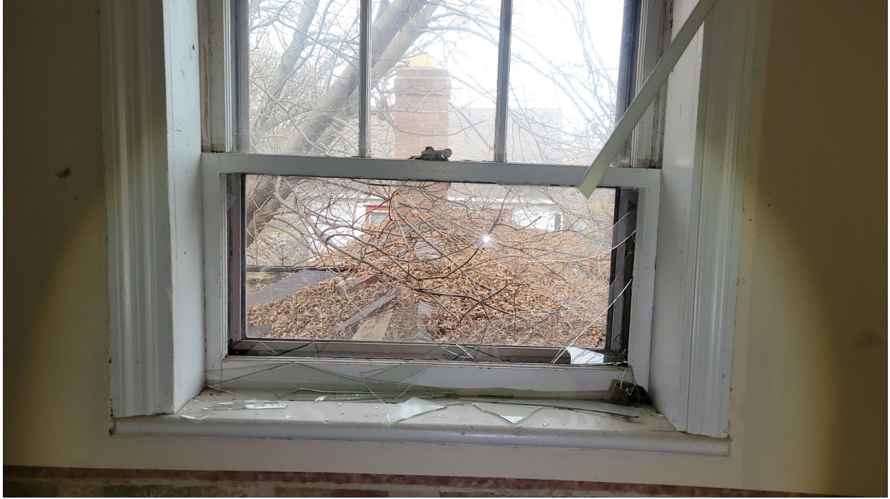
Photo 119: Replace all windows on Second floor that are broken.
