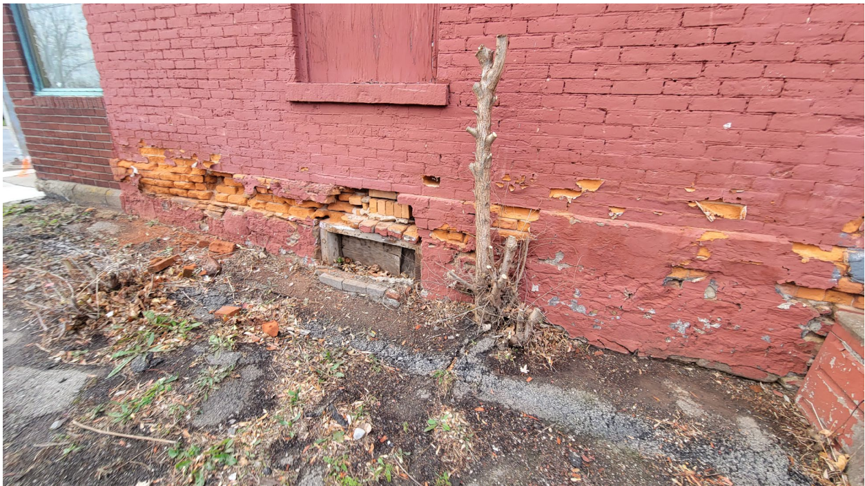
Photo 174: Repair and repoint all exterior brick.
