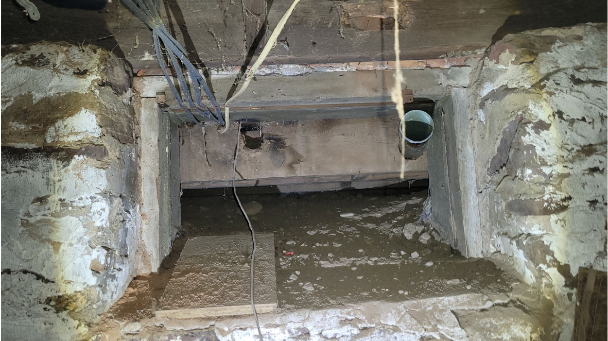
Photo 19: It is recommended that all window openings in the basement be replaced with glass block typically.
