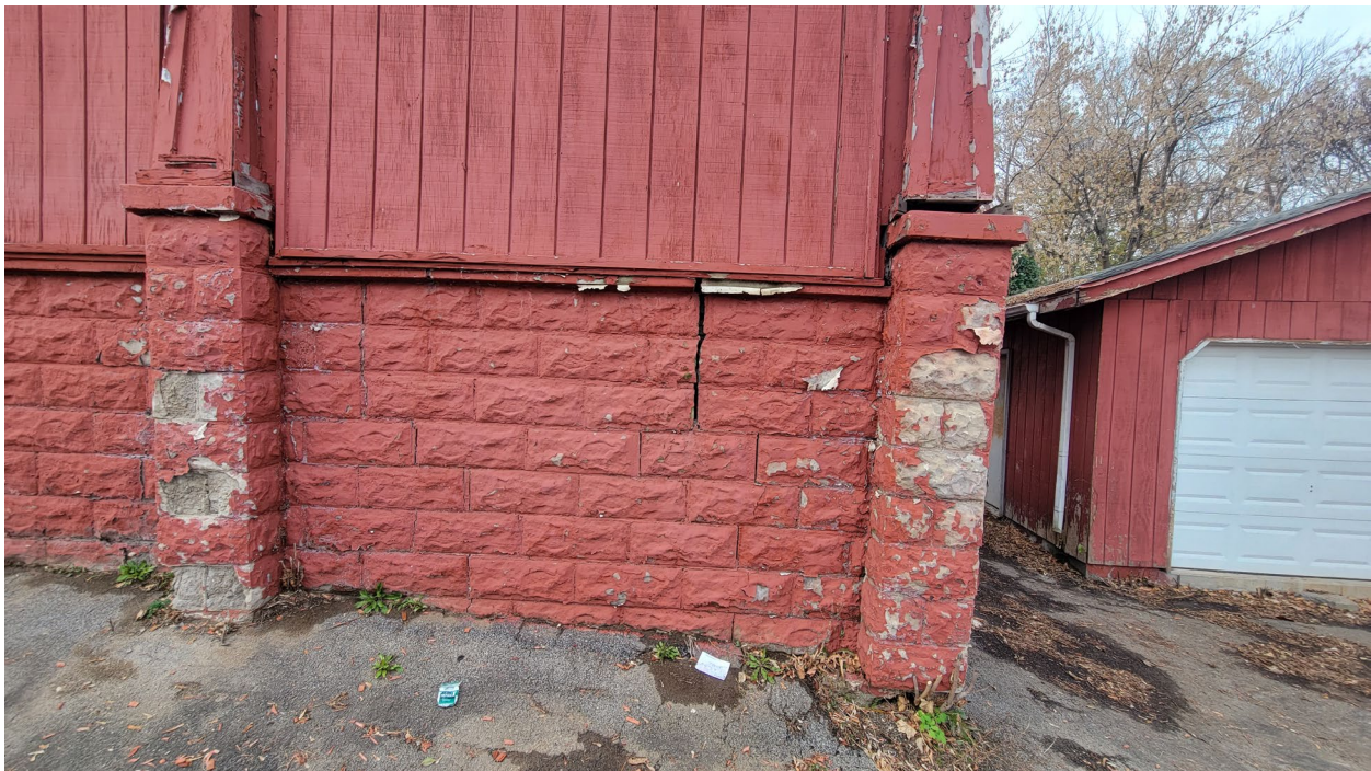
Photo 168: Evidence of settlement. It is recommended to seal the cracks with a non-shrink grout and then seal the face of the crack lines with an epoxy sealant. Monitor if there is any crack propagation over the next 6 months. If cracks return, contact the Engineer (Grefrath, 716-491-0019) for reinforcement recommendations.
