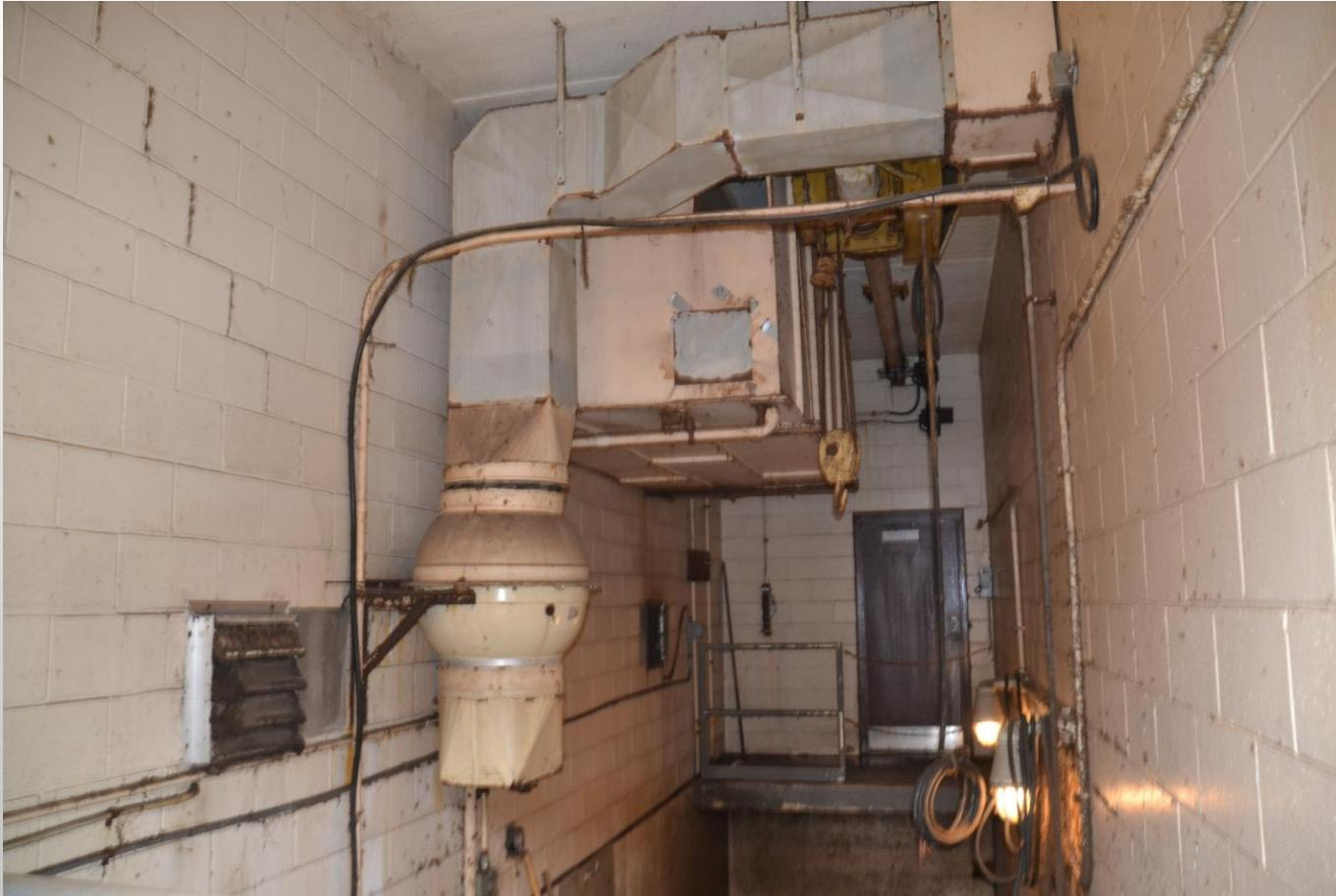
***Corrosive atmosphere due to hydrogen sulfide
