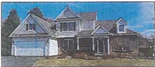
WEST FACE LOOKING EAST
