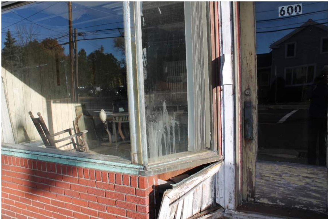
Photo 13 – View of asbestos containing window caulk on the copper window frame on the storefront windows, front of building.
