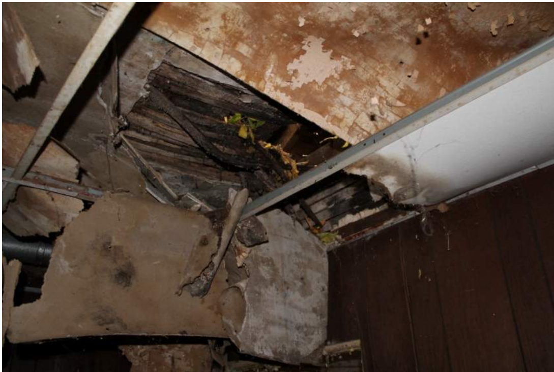
Photo 8 – View of wall panels with asbestos-containing mastic on the first floor. Note: Dangerous site conditions, ceiling collapsed.
