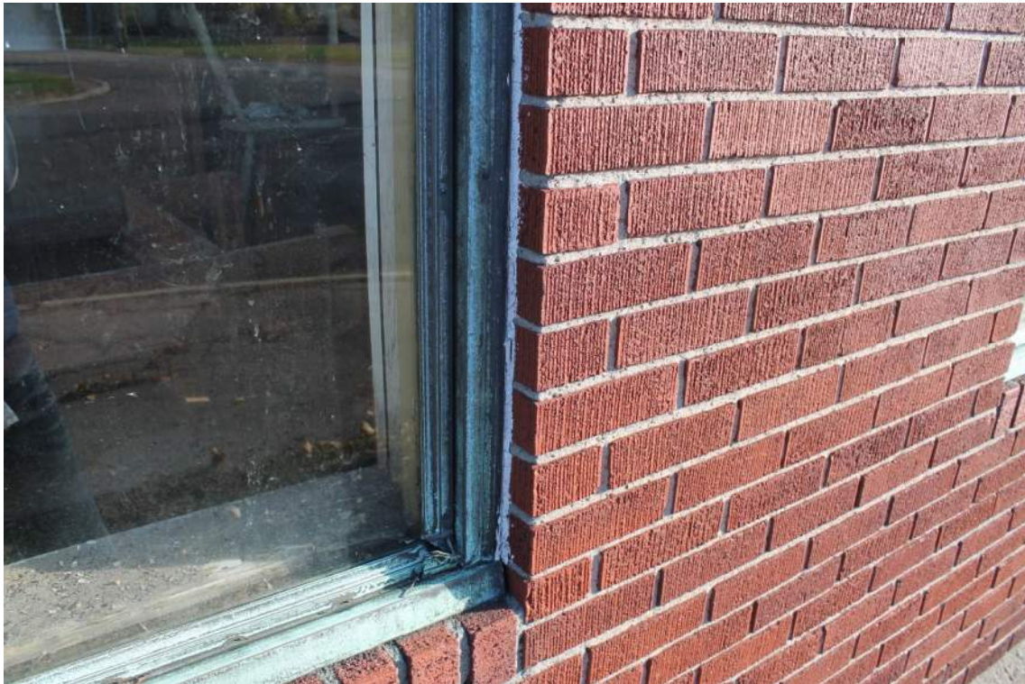
Photo 11 – View of asbestos containing window caulk copper frame to brick on the exterior storefront windows.
