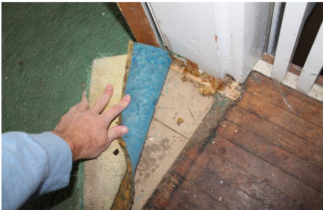
Photo 9 – View of asbestos containing 9 x 9 pink floor tile and associated black floor tile mastic under carpet in the second-floor apartment.
