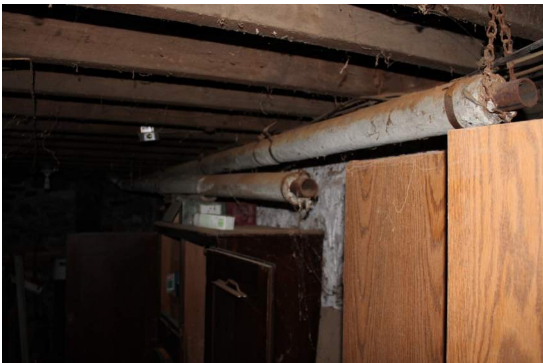
Photo 6 – View of asbestos-containing pipe insulation in the basement. Assumed present in wall cavities on the first floor.
