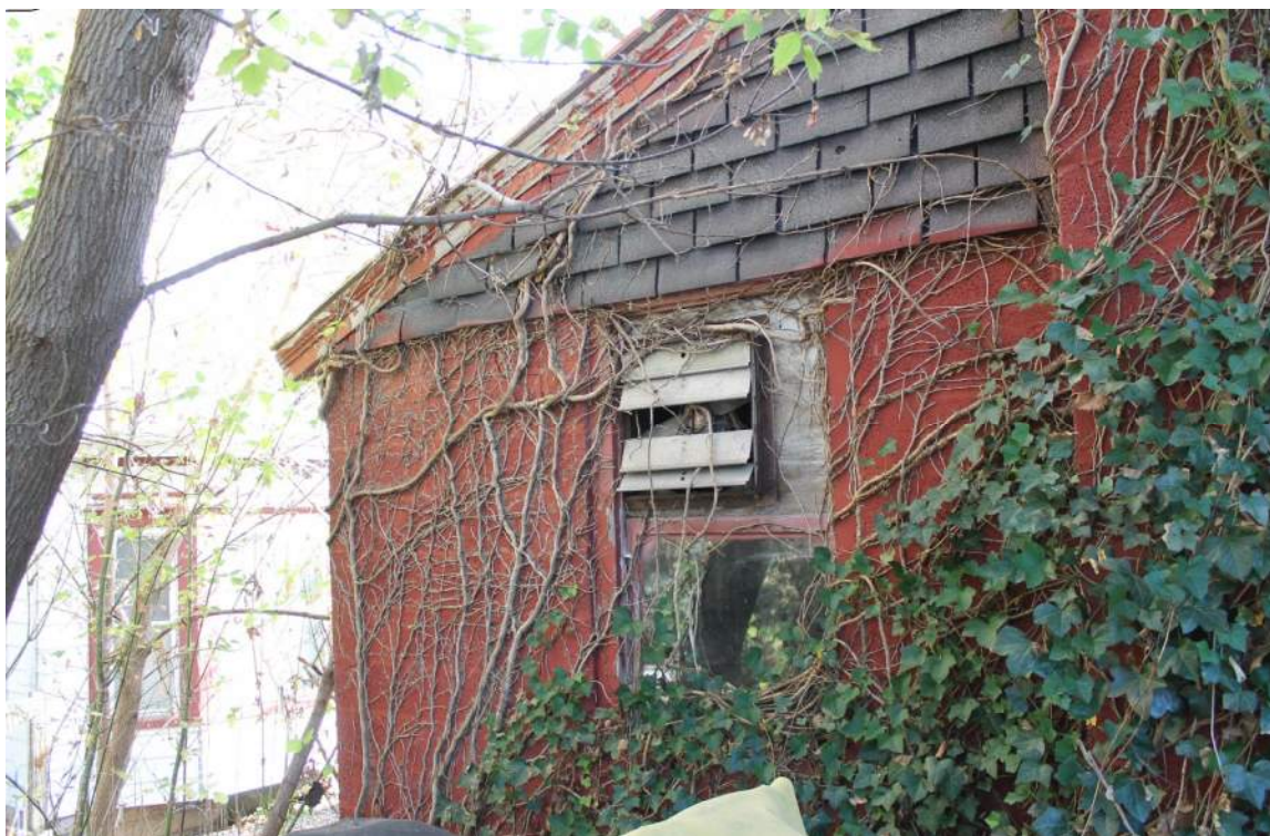
Photo 12 – View of asbestos containing window glazing compound on exterior garage window.
