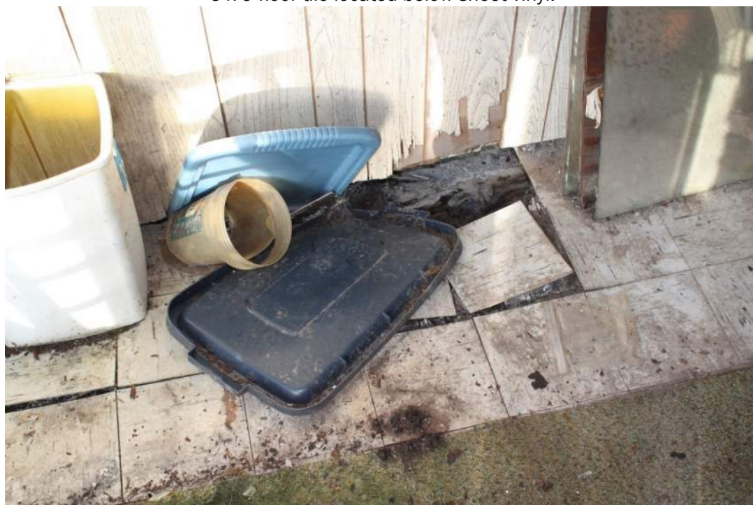
Photo 4 – View of asbestos-containing 9"x 9" white floor tile and associated black floor tile mastic on the first floor.
